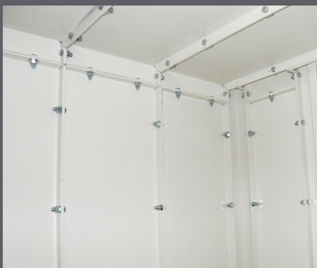
3/16" THICK STEEL WALLS AND CEILING
